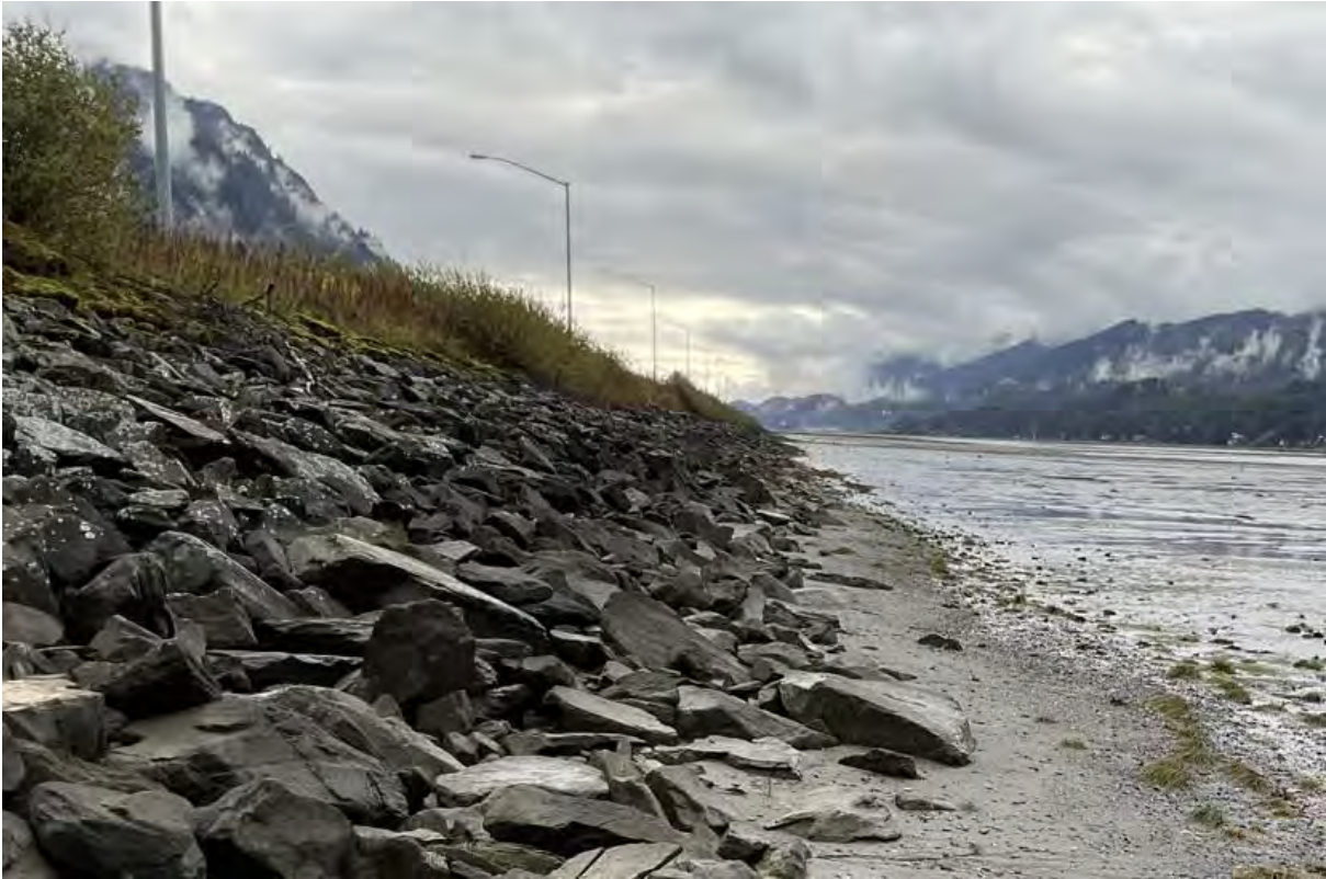
Riprap bank armoring along Gastineau Channel in Survey Area A9, facing south.
