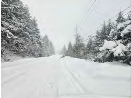
D. N. DOUGLAS HIGHWAY FACING NORTHWEST (January 2024)
