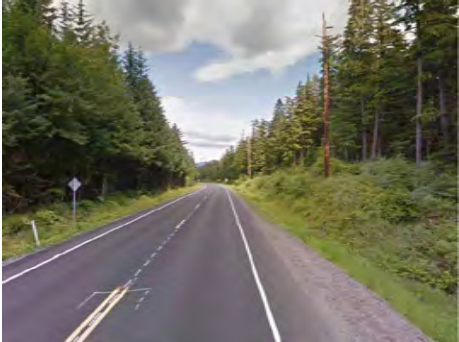
C. N. DOUGLAS HIGHWAY FACING NORTHEAST (Google Earth 2023)
