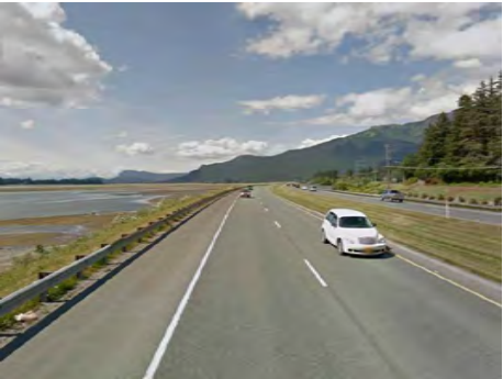
B. EGAN DRIVE FACING NORTHWEST (Google Earth 2023)
