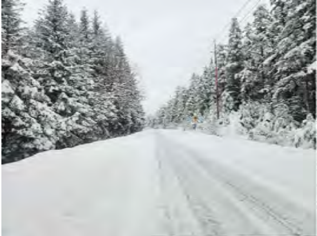
C. N. DOUGLAS HIGHWAY FACING NORTHEAST (January 2024)
