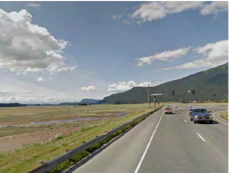
B. EGAN DRIVE FACING NORTHWEST (Google Earth 2023)
