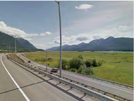
B. EGAN DRIVE FACING NORTHWEST (Google Earth 2023)
