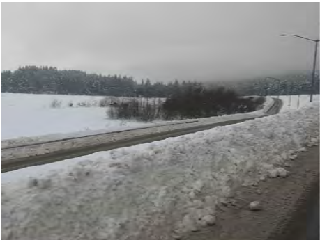
A. EGAN DRIVE FACING SOUTHEAST (January 2024)
